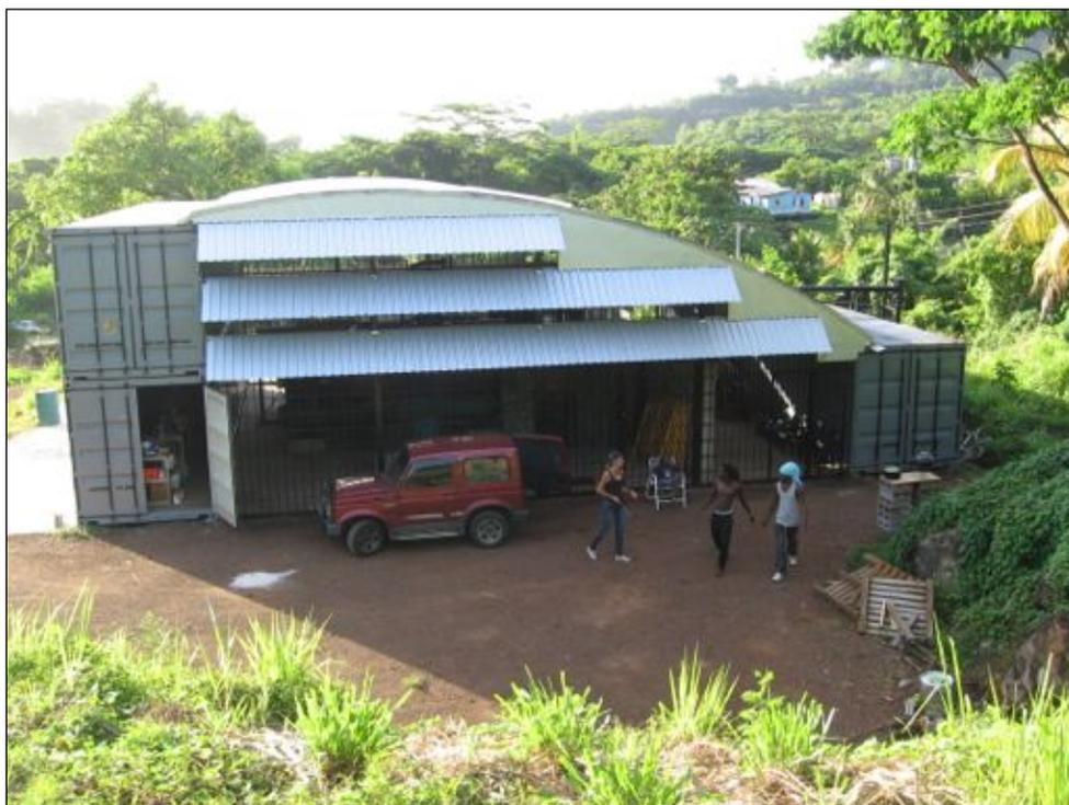
This is the new PFW plant. The building was assembled with a U.S. made prefab roof and the original containers used to ship the machinery overseas. The plant is designed to provide flow through ventilation so that the elevated temperatures created in the manufacturing process can quickly escape protecting the workers from unnecessary heat stress.
